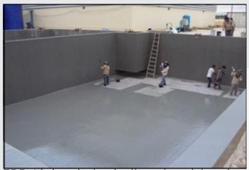
FRP Lining is basically a hand lapping process where Glass Fiber used with different type of resins as per the chemical compositions and type of exposure. The basic advantages of FRP Lining the application are very simple along with the surface preparation required before the application. It does not required the tedious process of sand blasting as in other linings required. And we can select the resin as per the job applications and the cost also varies accordingly.
